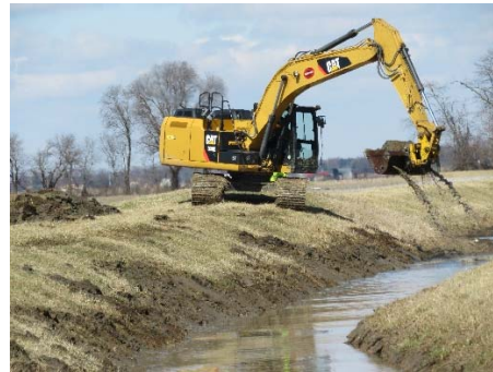
PCE crews cleaning Greenbriar Ditch
