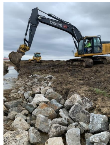
Regrading work on Audi Howard Ditch
