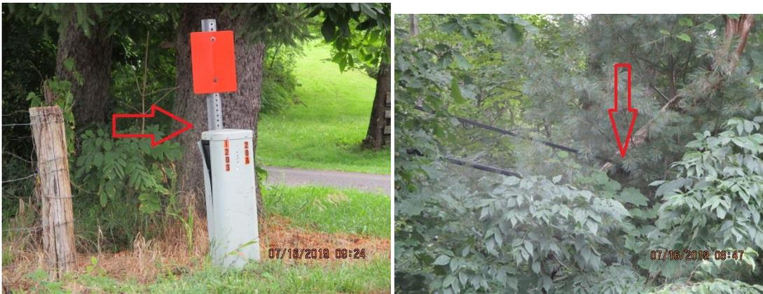
68. The above pictures show a damaged pedestal at the road near the lane to the BLES customer's house and a large tree limb on a cable near a customer's property in Carroll County.
